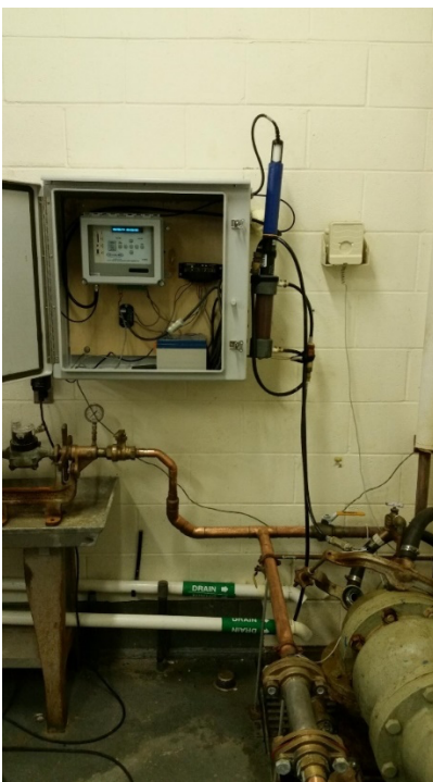
Figure 19 – Example of well pump house instrumentation of for measuring in-situ groundwater quality properties.
