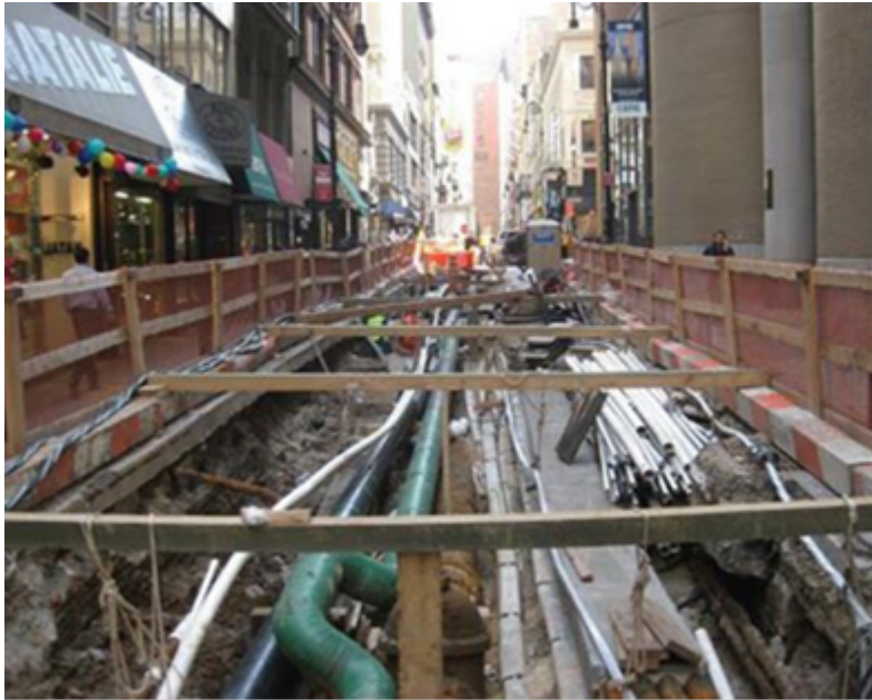
Figure 7. Lower Manhattan Utility Excavation (NYC Office of Emergency Management)
