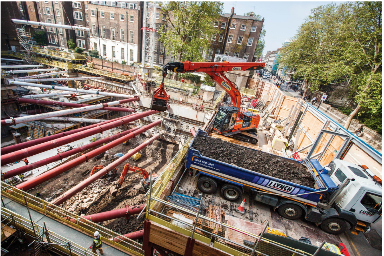
Figure 27. Rare view of underground network infrastructure minus the usual surrounding earth and built materials
